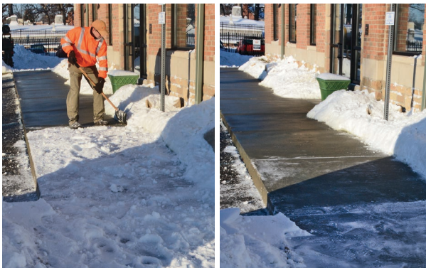
Shoveling and bare surface results are achieved easier after pretreating with liquids.
