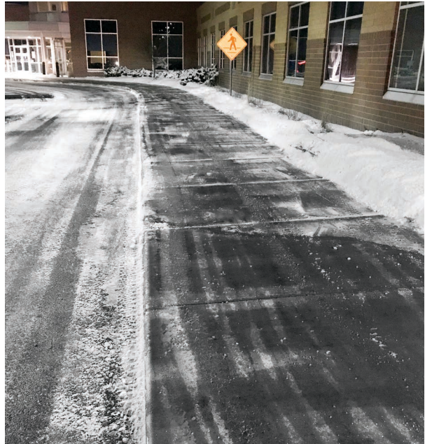
A salt brine blend can be used as a post-treatment, even at sub-zero temperatures.
