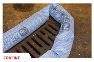
Set up absorbent socks (overlap ends) to contain the spill and prevent it from flowing any farther or into waterways. If available set up a fluid collection container to collect dripping or running fluids. Next, if available, use a patchand-plug product to stop the leaking/dripping at its source.
